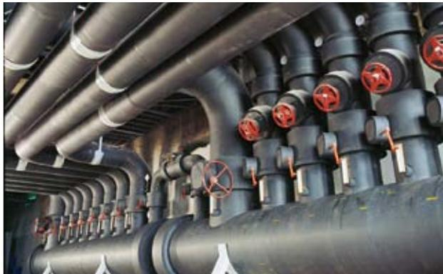
Many advantages described above making Aeroflex suitable for insulating chilled water piping.
