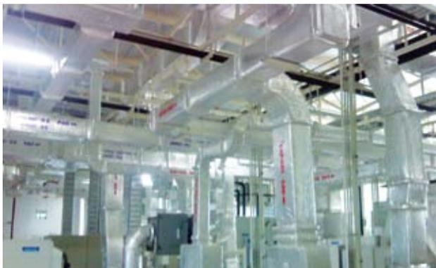
Neat appearance when used as external insulation for air ducts in phamasutical laboratory facility.
