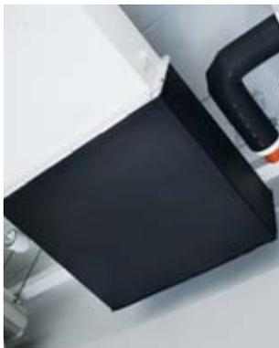
Aeroflex can work efficiently as an sound dampening material when used as internal and external insulation for medium and high velocity air duct system.
