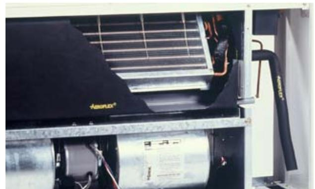
Aeroflex does not contain any fibrous material, so it is safe to use in direct contact with air, provides the excellent IAQ (Indoor Air Quality) Standard.
