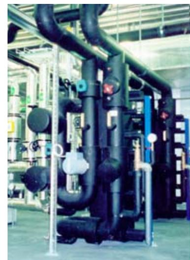
*Because of low water absorption and water vapor transmission, Aeroflex is widely used in heating and cooling system.*
