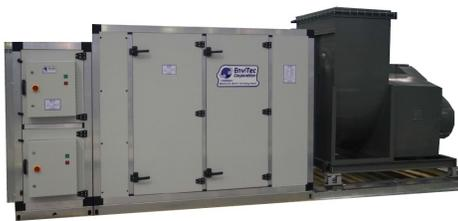
EAPU with Externally Mounted Fan
